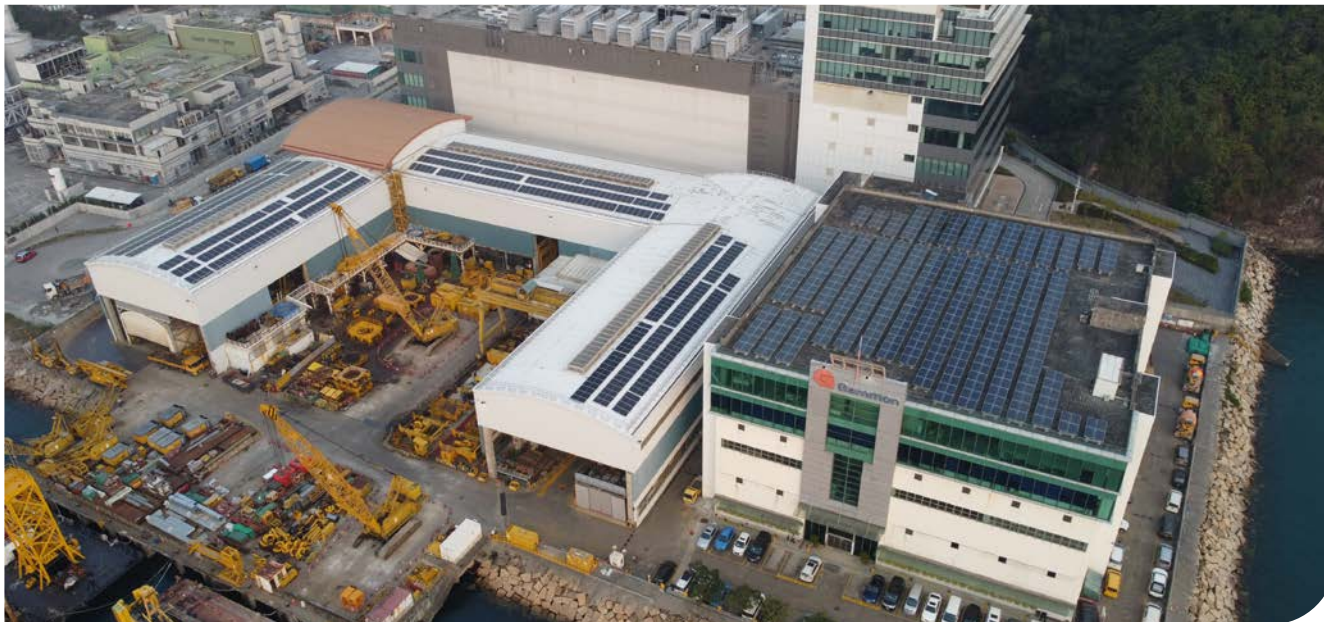
400 kW capacity solar installation at Gammon Technology Park in Tseung Kwan O
