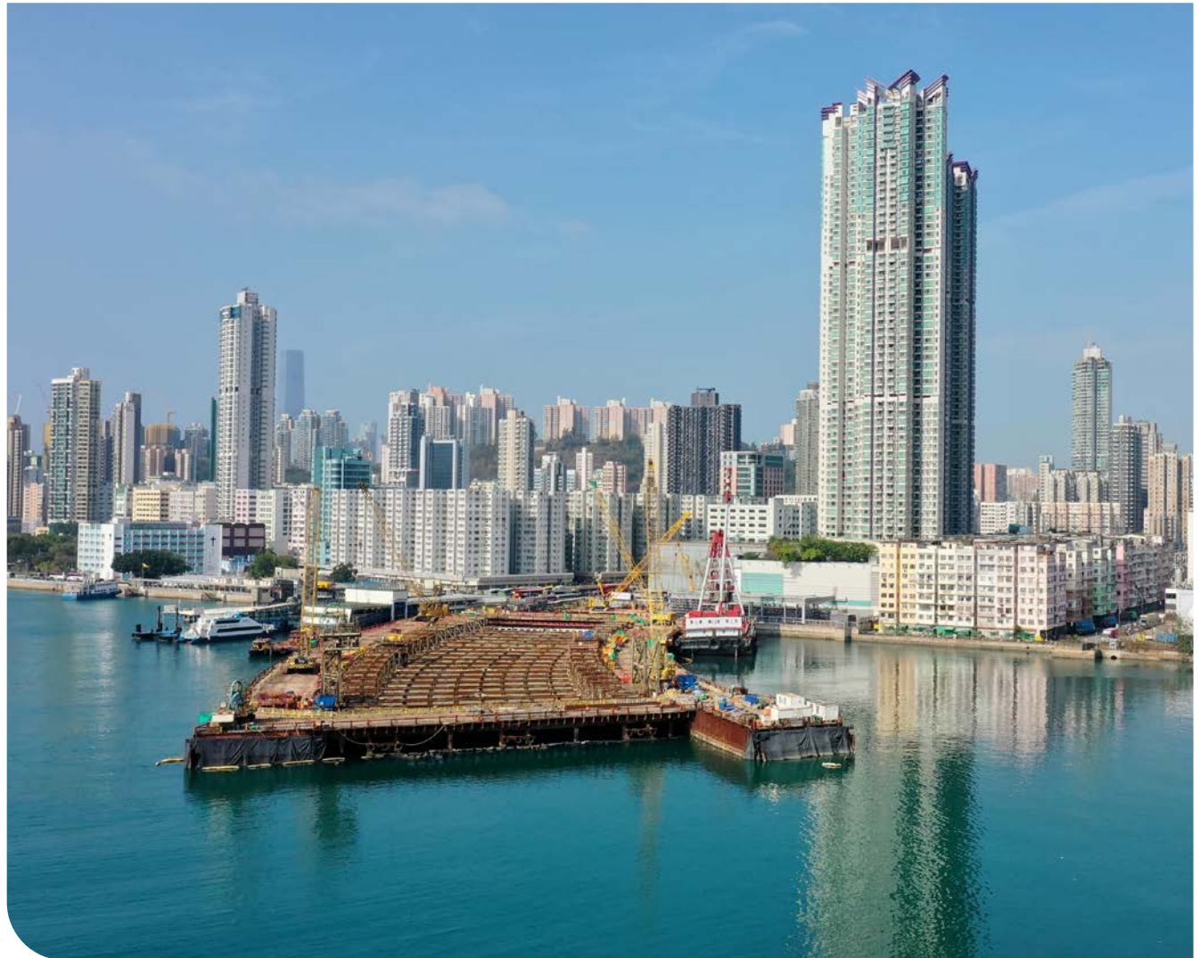
Modular steel struts such as those from our Central Kowloon Route - Kai Tak West contract are being re-used on other projects
